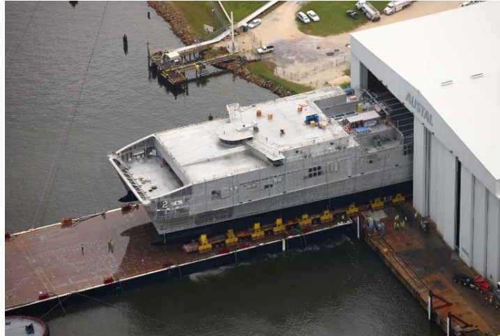
FIGURE 2-1 JHSV BEING MOVED ON SPMTS
